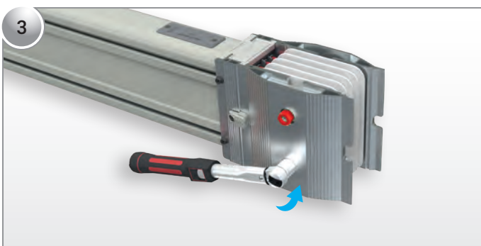
Loosen the block joint nuts.
